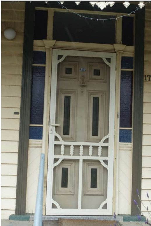
Figure 14. Original six-panel front door at No. 17. Note the pressed glass and diagonal boarding below sidelights. (Landmark Heritage 2022)
