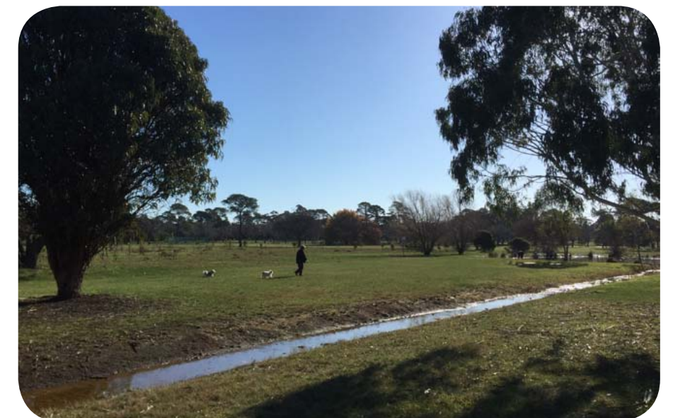
Existing open swale outlet drain
