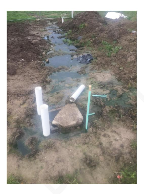
Figure 3: Example of septic effluent emerging in the backyard of a newly constructed house in Bonshaw, July 2016. Both houses were in the Declared Sewer District. The effluent originated from the septic of a house located 70m away which had not been inspected or mapped. Emergency sewer works had to be completed at considerable time and expense for City of Ballarat and Central Highlands Water.
